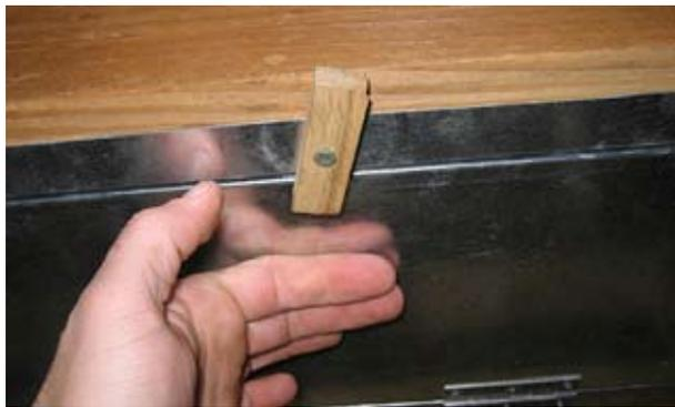
During visits in the field, we often see houses where inlets are opening only about 1/4 inch. This small an opening will not produce high velocity air and will result in very poor air mixing. Poor air mixing results in chilled birds, wet floors and high fuel costs.
