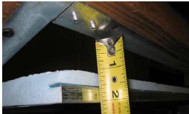
An inexpensive latch or nail to seal off unneeded air inlets is perhaps one of the best tools in setting up houses for good winter airflow. The number of inlets to be used must be matched to number of fans that will come on. During brooding and cold weather, a large number of the inlets must be closed off to assure good airflow.
