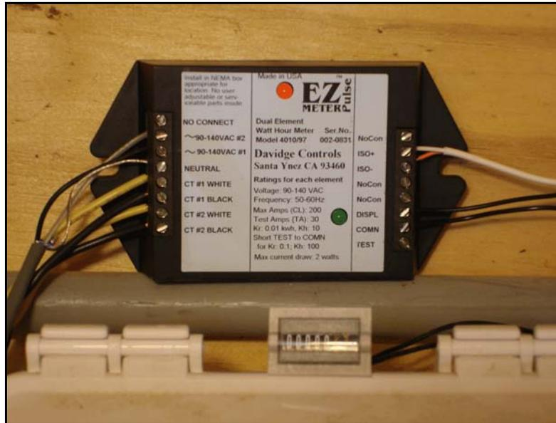
Figure 1. Power (Kw\*hr) meter with optional mechanical display.
